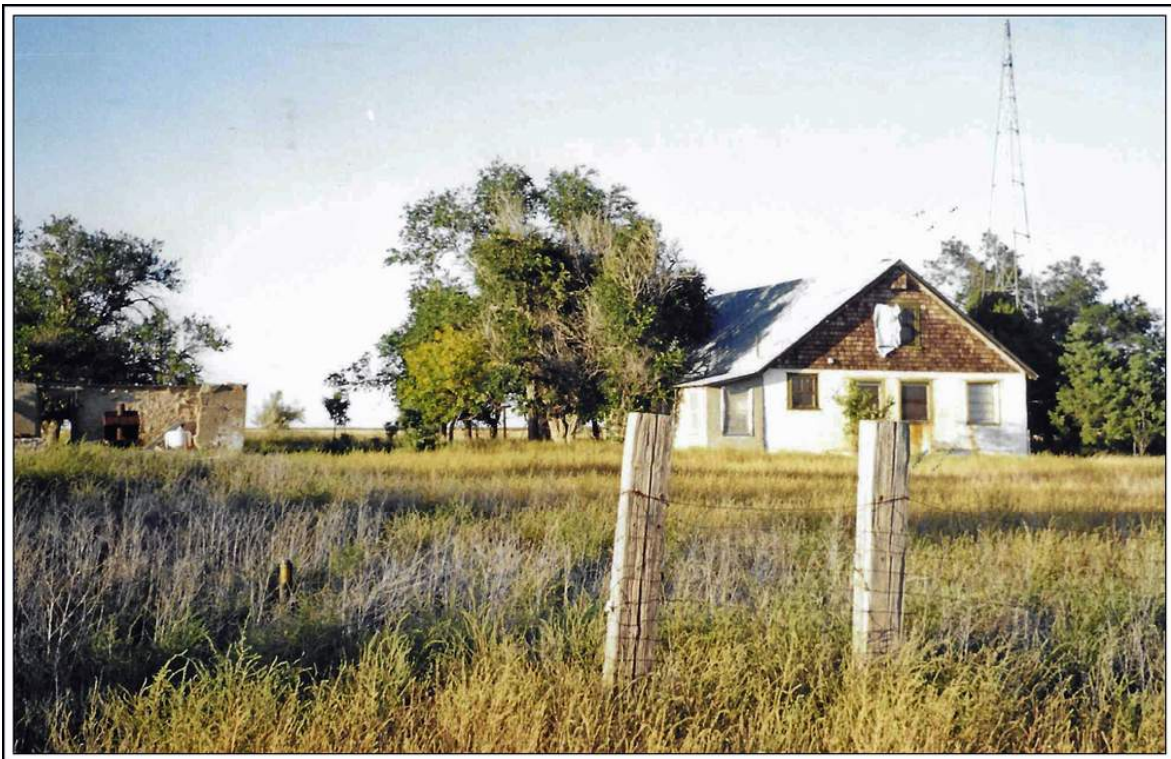
Ranch buildings at the site of Zuck, Colorado
