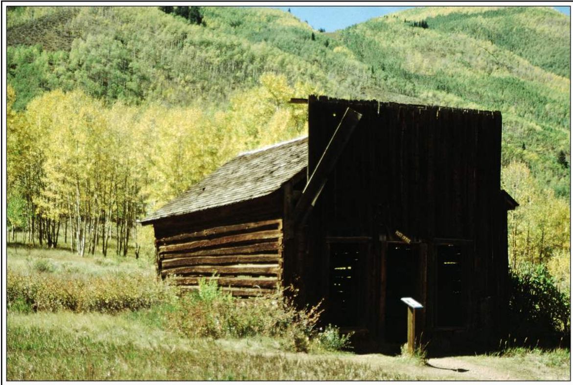
This stabilized log building at Ashcroft is identified as the post office. Photograph by William H. Bauer September 16, 2002
