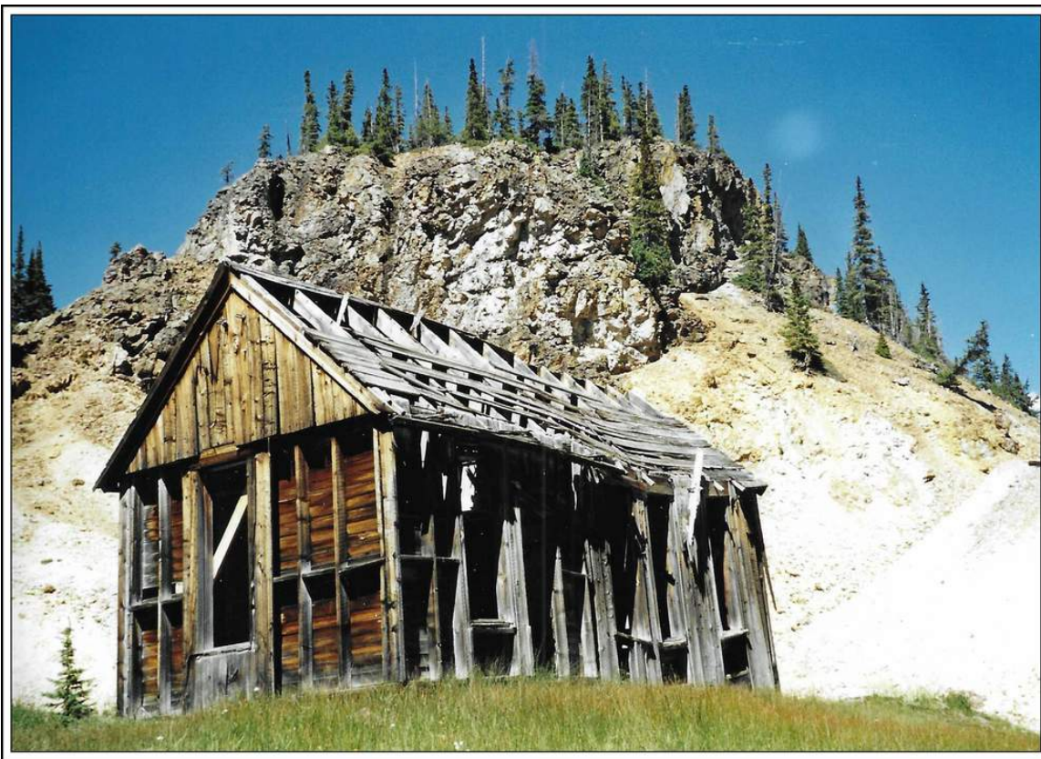
The remaining building of the National Belle Mine at Red Mountain, Colorado Photograph by William H. Bauer August 25, 2004
