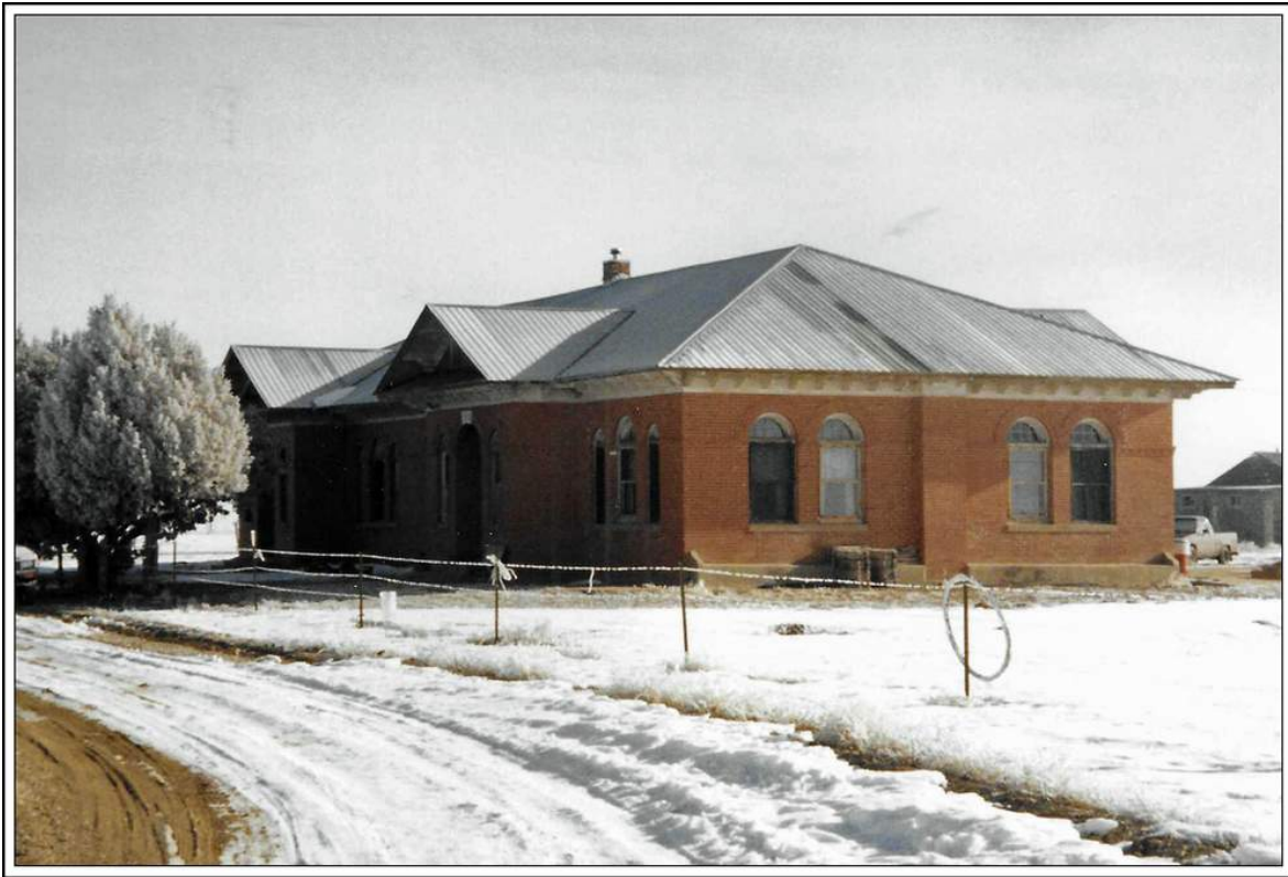
Timpas, Colorado – Formerly a school, this building is now a private residence.
