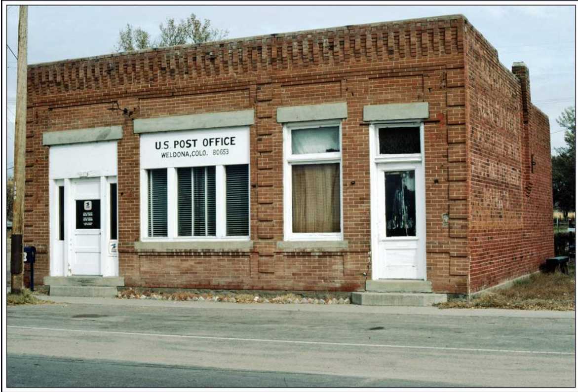
This building once housed the post office at Weldon, Colorado.
