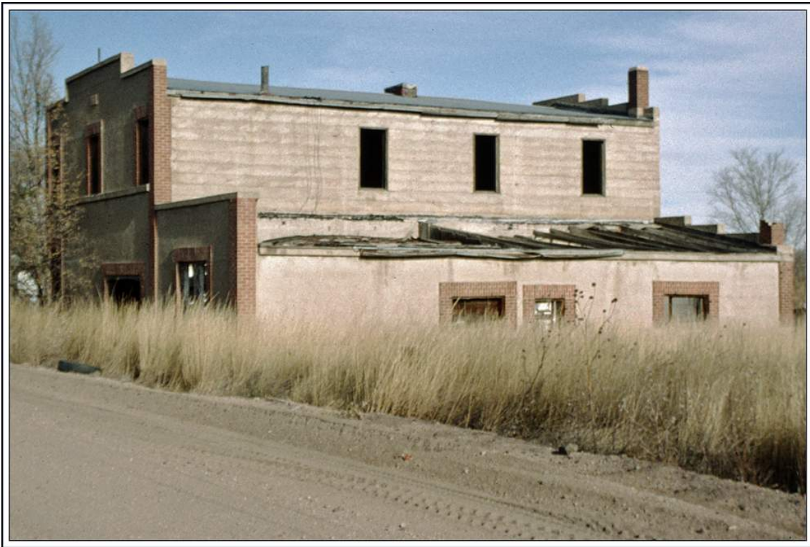
This abandoned building at Pawnee, Colorado has the appearance of having been a store.
