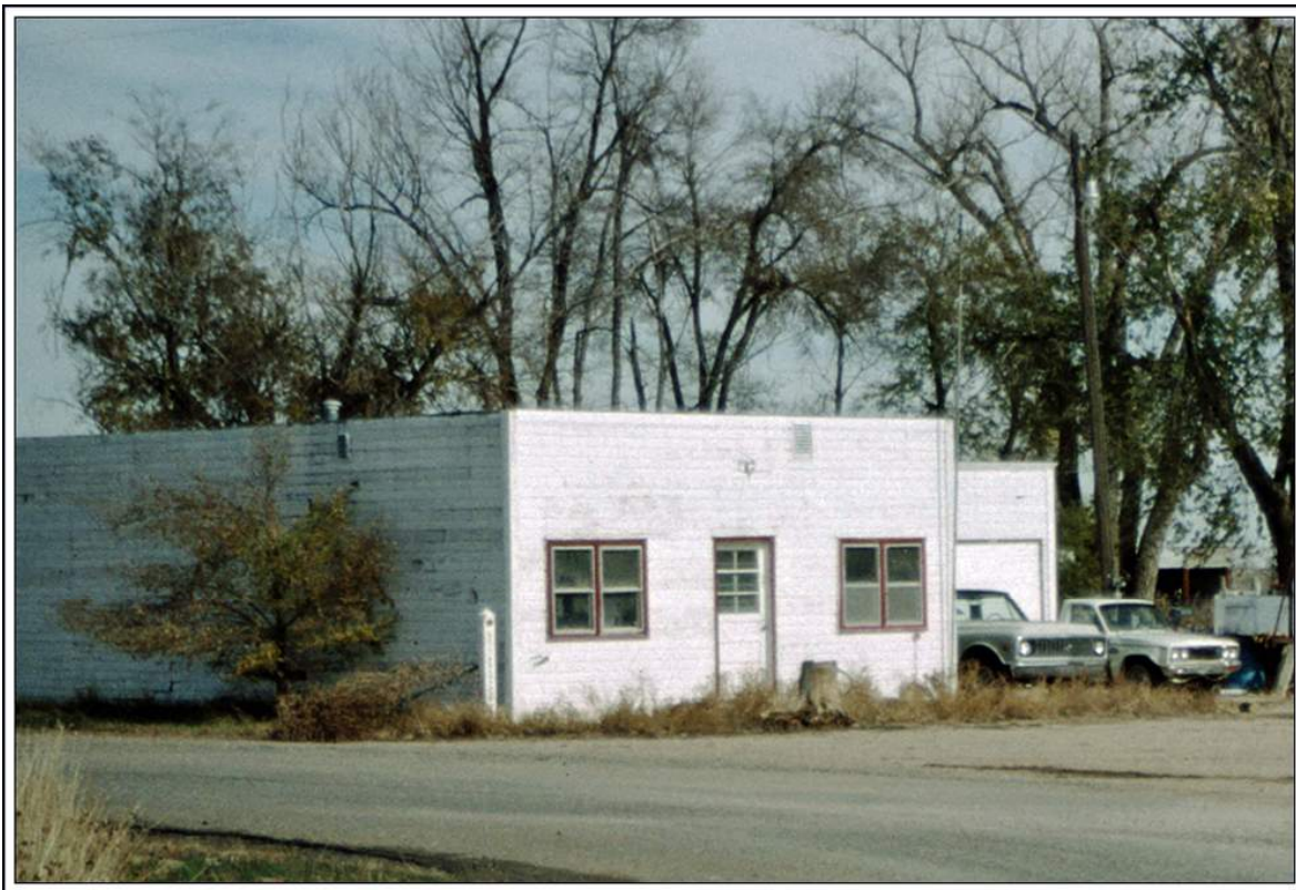
Hoyt, Colorado – This building was the final location of the Hoyt Post Office. Photograph by William H. Bauer November 8, 2005
