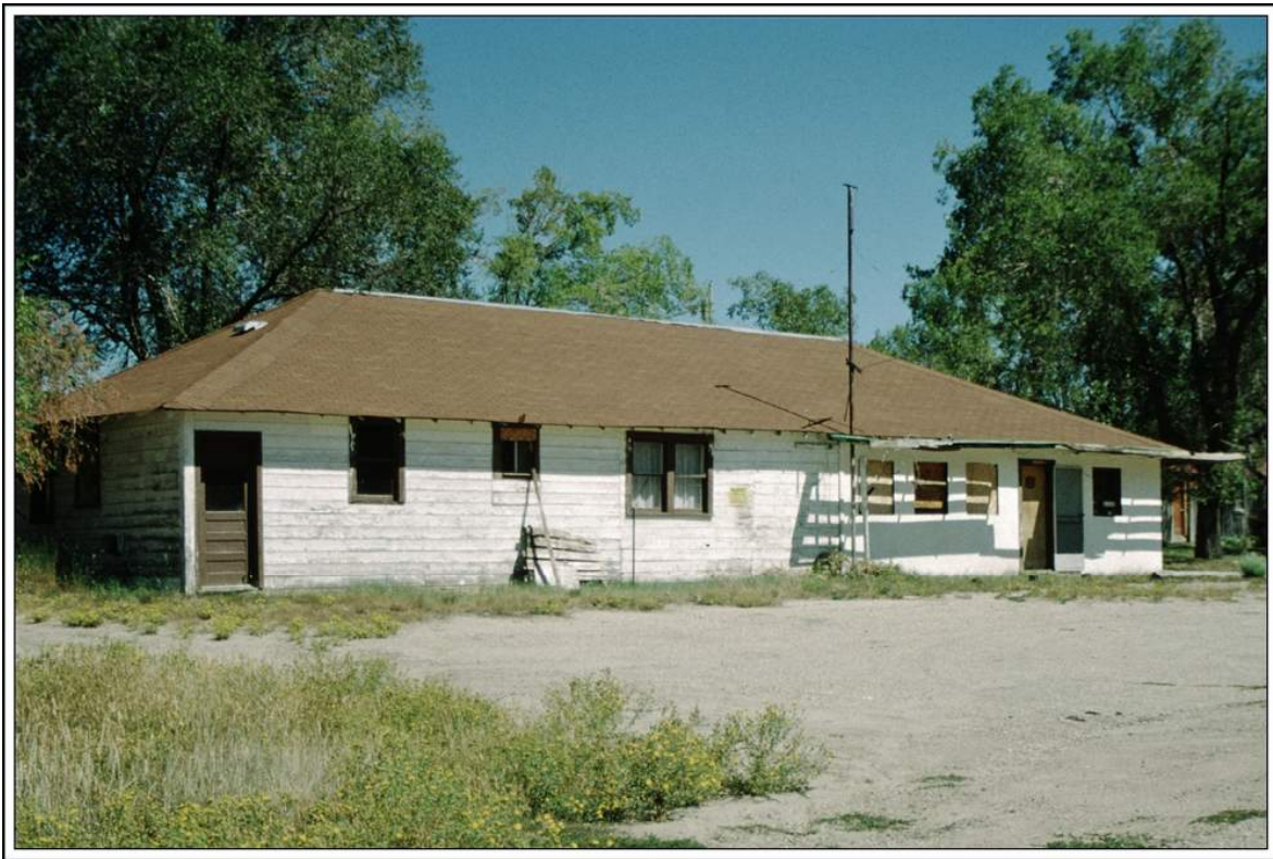
This building once housed the Elk Springs Community Post Office and a café. Photograph by W. H. Bauer September 2, 1998
