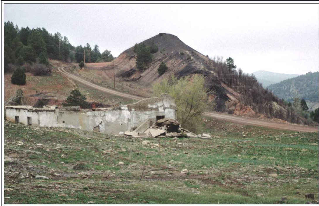
Foundations and mine dump at the site of Morley, Colorado Photograph by William H. Bauer May 7, 2001
