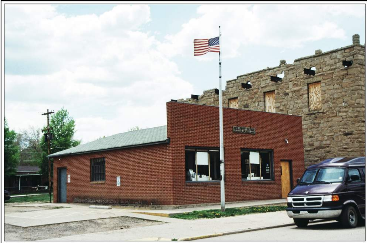
Post Office – Aguilar, Colorado Photograph by William H. Bauer May 10, 2001
